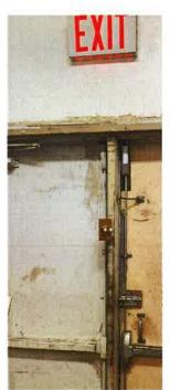
There is evidence in town of improper Fire Door maintenance. Fire exit doors are not permitted to have any barrel bolts, chains, L-hook or any other latching appliance except the one door latchina mechanism. This is defined by the National Fire Code Alberta Edition 2.7.2.17 and the National Building Code Alberta Edition.
